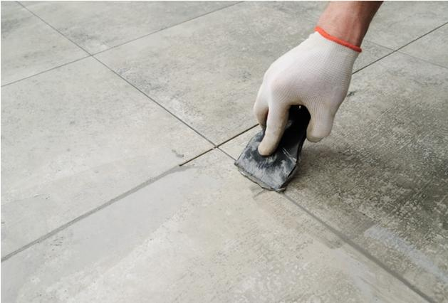
12. Epoxy based joint fillers should be chosen in places with heavy pedestrian traffic.
