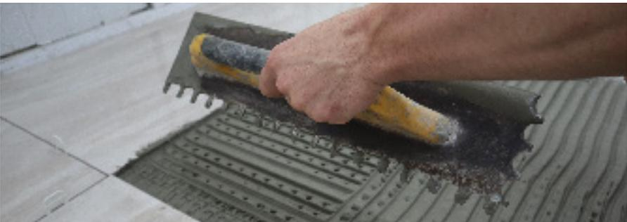
9. In all applications, the adhesive must be bonded after the adhesive has been applied to both the surface and the back of the tile. Adhesives should contact the back of the tile 100%. In order for the adhesion to be strong and for the adhesive to fully spread and adhere to the back of the tile, the tile should be tamped lightly with a rubber mallet.
