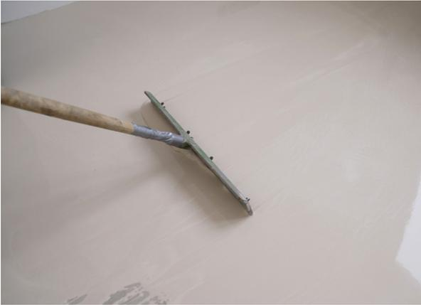
4. The floor or wall where the ceramic will be laid should be smooth, if there are curvatures, level differences, should be corrected with suitable screed material beforehand, if there are drains on the floor, the desired slope towards the drain should be calculated and this angle should be applied with the disposal screed.
