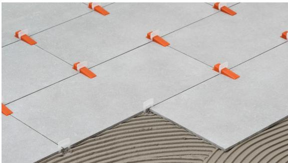
17. For products with an aspect ratio of more than 2 times such as 30x120 ( $120/30 = 4$ ), as we have stated in the product boxes, the applications should be made in a 1/3 ratio. Information on the box is as follows. This means that for a product with a long side of 120 cm, it is tiled with a shift of  $120 \text{ cm} * (1 / 3) = 40 \text{ cm}$ .
